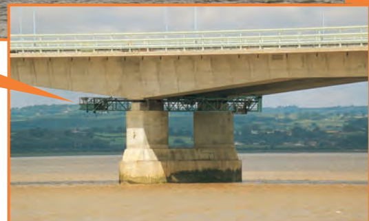
Access Gantry on Second Severn Bridge
