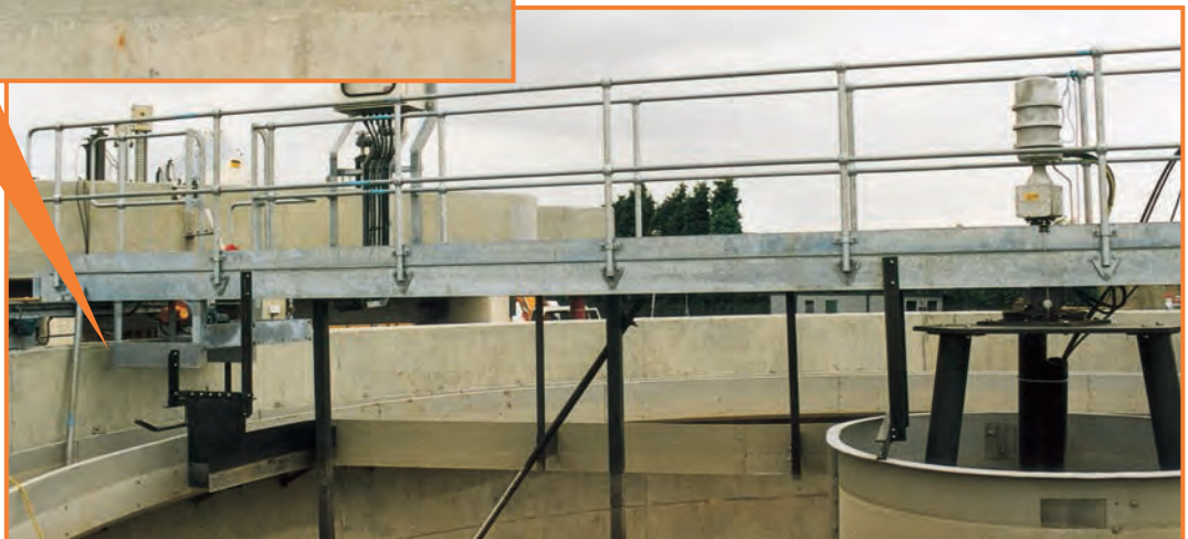
Half Bridge scraper for rotary settlement tank
